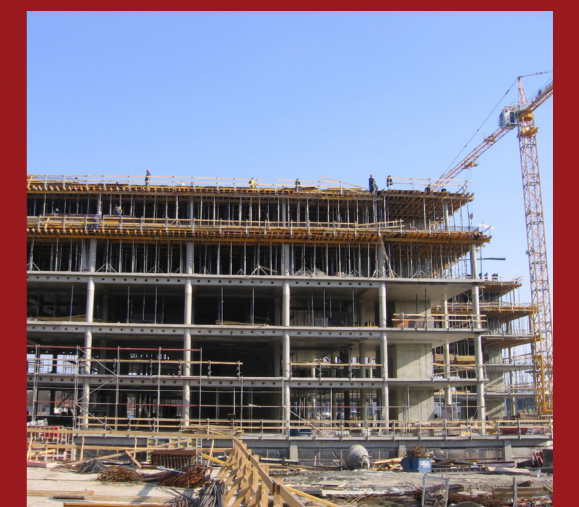
Baneasa Business and Technology Park
